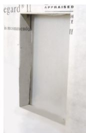
Apply weather proofing
