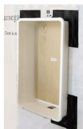
Fix meter box in place
