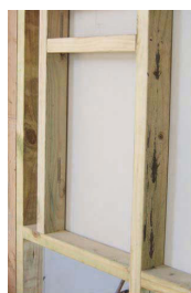
Frame to fit meter box
